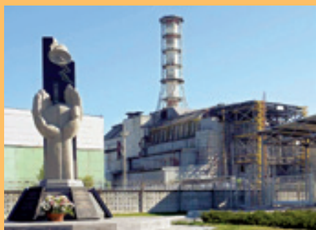
Reactor 4 in Chernobyl, which exploded in 1986, is enclosed in a sarcophagus of concrete, whose west wall has recently had to be supported with a steel frame.
