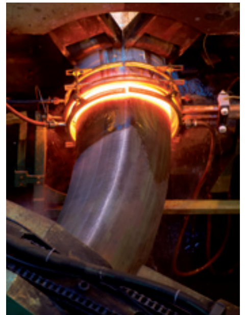
Using the induction bending process, pipes in diameters of 114.3 to 1,625.6 mm are bent through up to 180 degrees
