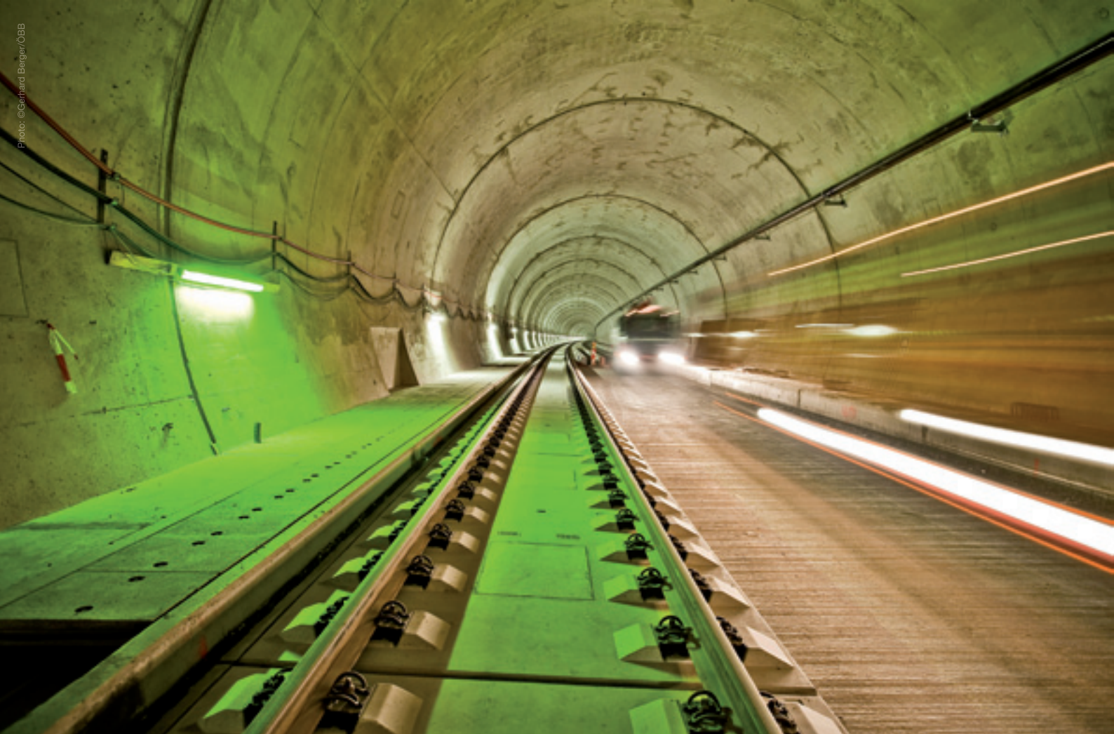
The tunnel during track-laying work
