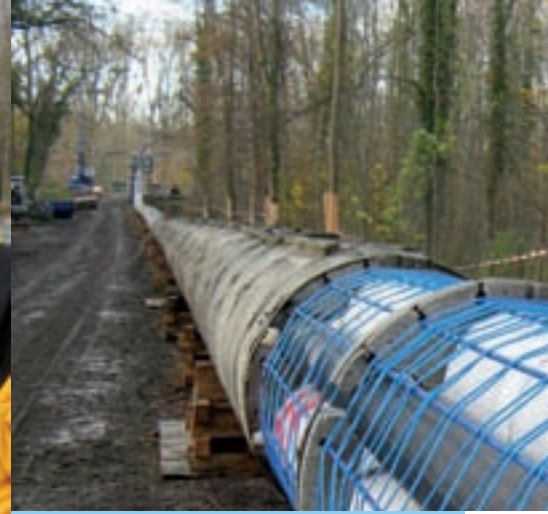
Left: Andreas Weishaupt, EPS Technical Manager, and Stephan Maier, Project Manager at Salzgitter Mannesmann Line Pipe, at the Rhine crossing near Karlsruhe. Top: Preparation of the underwater crossing. Underwater crossings are manufactured on land and then pulled into a river. One of the three pipe strings is already available in reserve for further projects.
