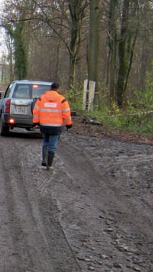
Preparing to cross the Rhine near Karlsruhe: The underwater crossing will be given a heavy coat of concrete before it can be finally pulled in.
