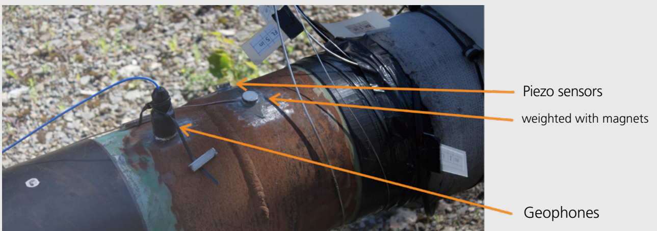
Figure 5: Fitting the structure-borne sound sensors
