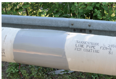
Cast field coating of cement mortar coated pipe joints
