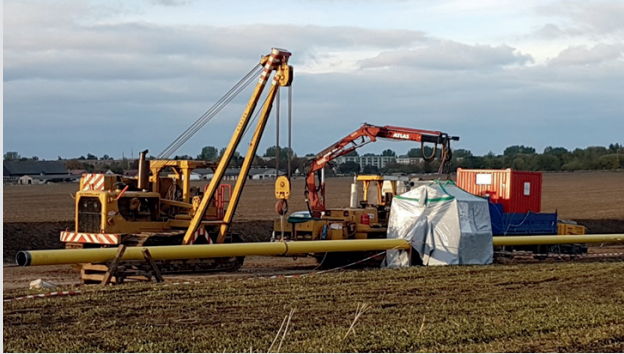
Figure 5: Construction site set-up
